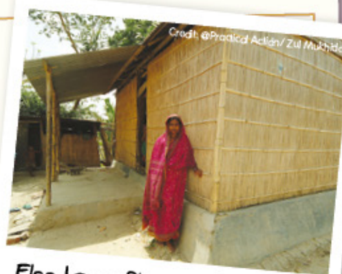
Flood proof home in Bangladesh
